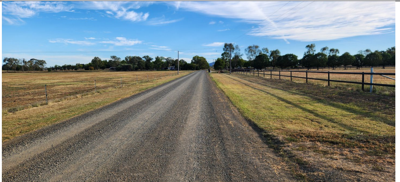
Figure 5 - Lot 2 - Access North
