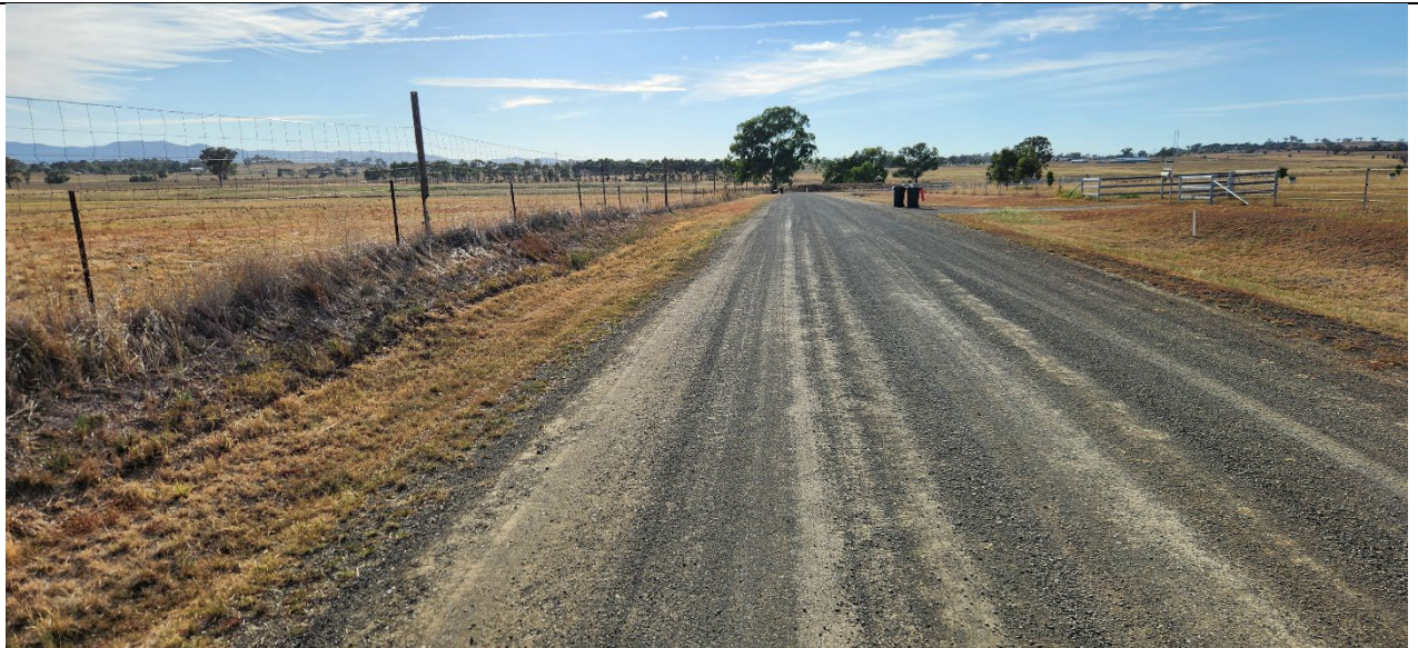
Figure 13 - Lot 4 - Access East
