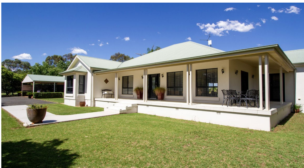
Figure 6 - Existing rendered dwelling with CBPM roof
