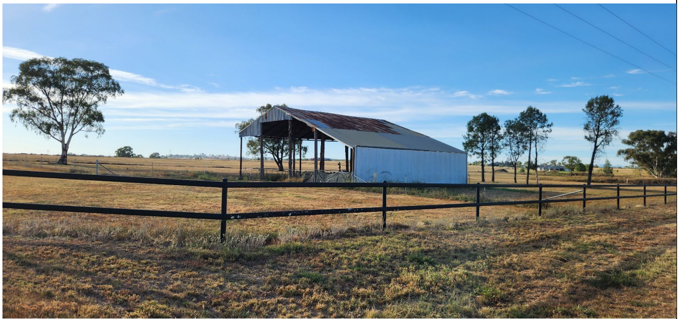
Figure 3 – Additional infrastructure example on site
